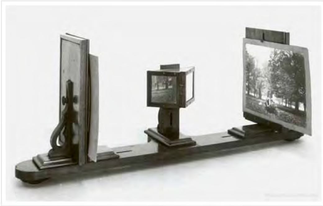
SIR CHARLES WHEATSTONE'S 'STEREOSCOPE,' 1838
